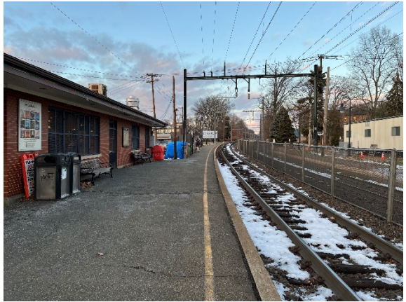
Photo 10: View east down Walnut Street platform
