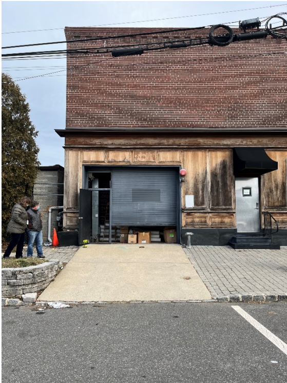
Figure 41: Loading area for 2 Erie on Label Street
