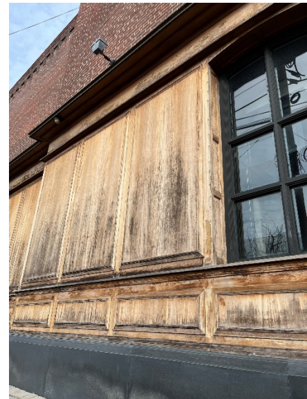
Figure 39: Wood paneling applied to first floor exterior
