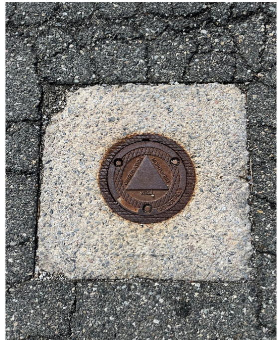
Figure 21: Groundwater contamination observation well
