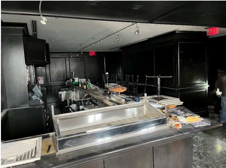
Figure 37: Interior of 2 Erie Street.
