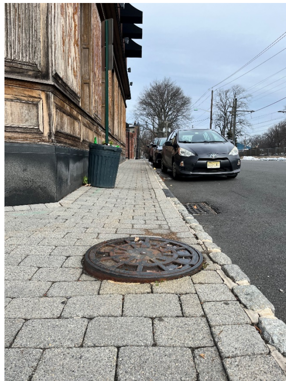
Figure 15: Underground stormwater utilities running beneath the sidewalk along Erie Street
