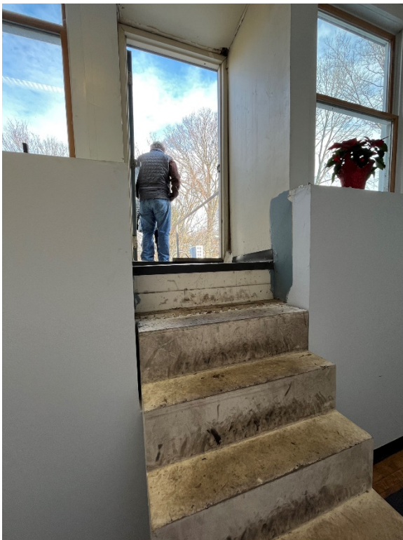
Figure 35: Egress stair to roof
