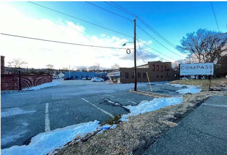
Figure 22: 4 Erie Street as viewed from the Walnut Street Station neighborhood platform
