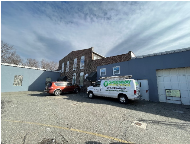
Figure 33: Exterior of 7 Oak Place
