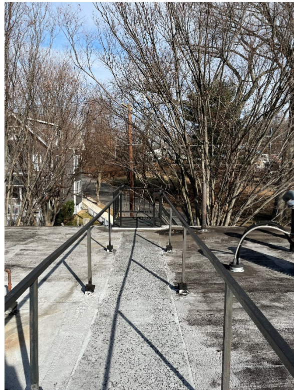
Figure 36: Roof access to fire escape
